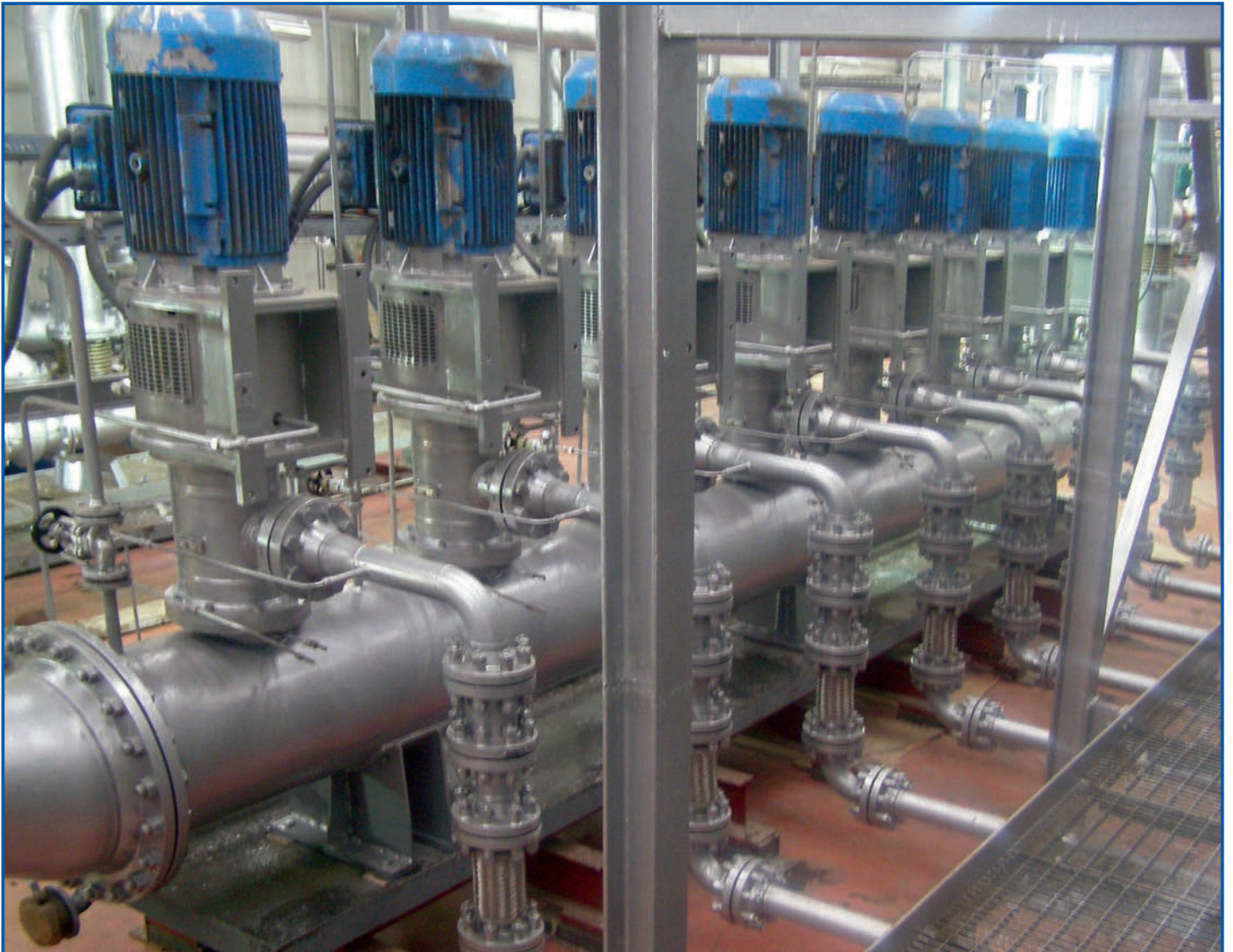
High pressure pump station prior to the work for the heat insulation
