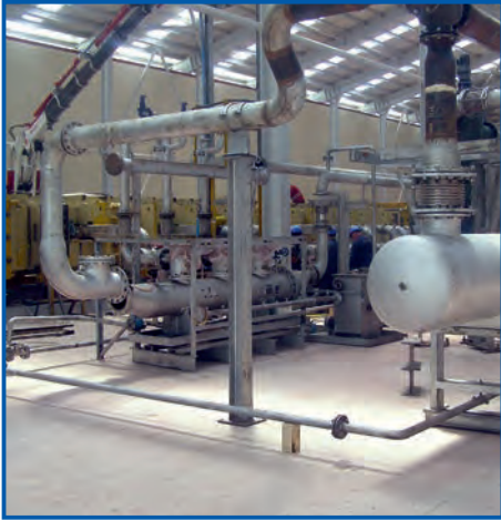
Start of the installation of the press and the components of the silicone oil circuits
