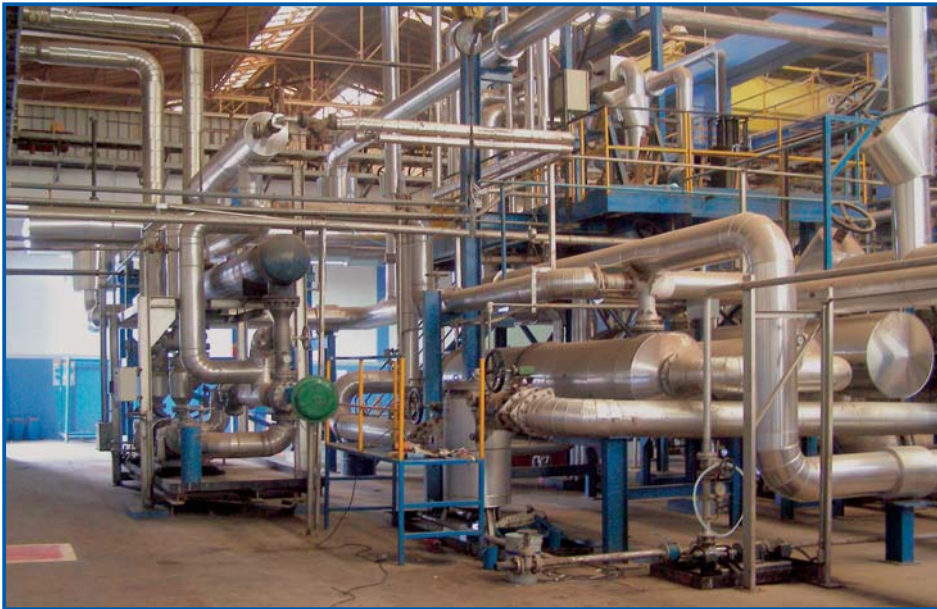
Heating/Cooling tubing section of press oil circulation system
