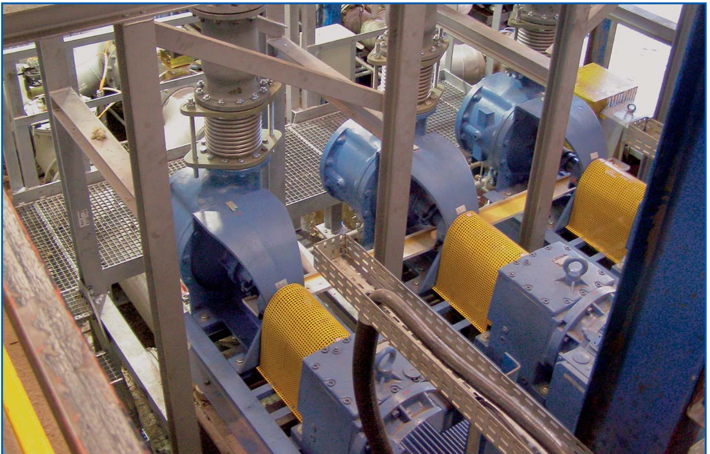
New gear type main circulation pumps of the press oil circulation system
